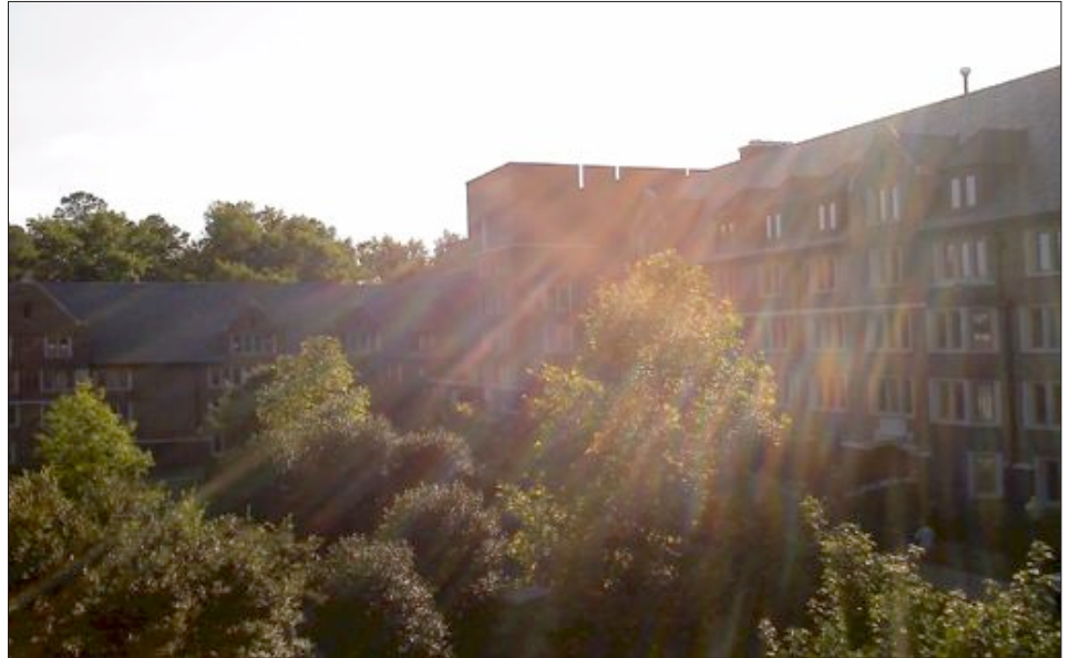
A new proposal would add beds to the Keohane quad, but at what expense?
